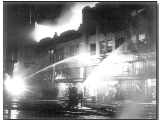
Figure 1-15 Whitney Department Store Fire
